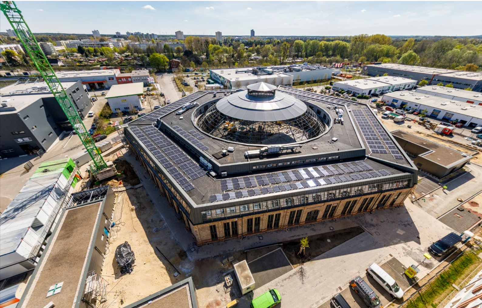
The hexagonal dome hall with a 20-metre-high Schwedler dome roof, which has a span of 48 metres, where solar panels are installed
